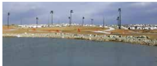
This photo shows Redstone Pond under construction in 1999.
